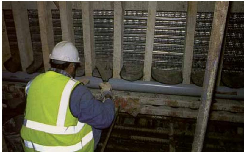
Example of *in situ* cast concrete showing expanded metal formwork
